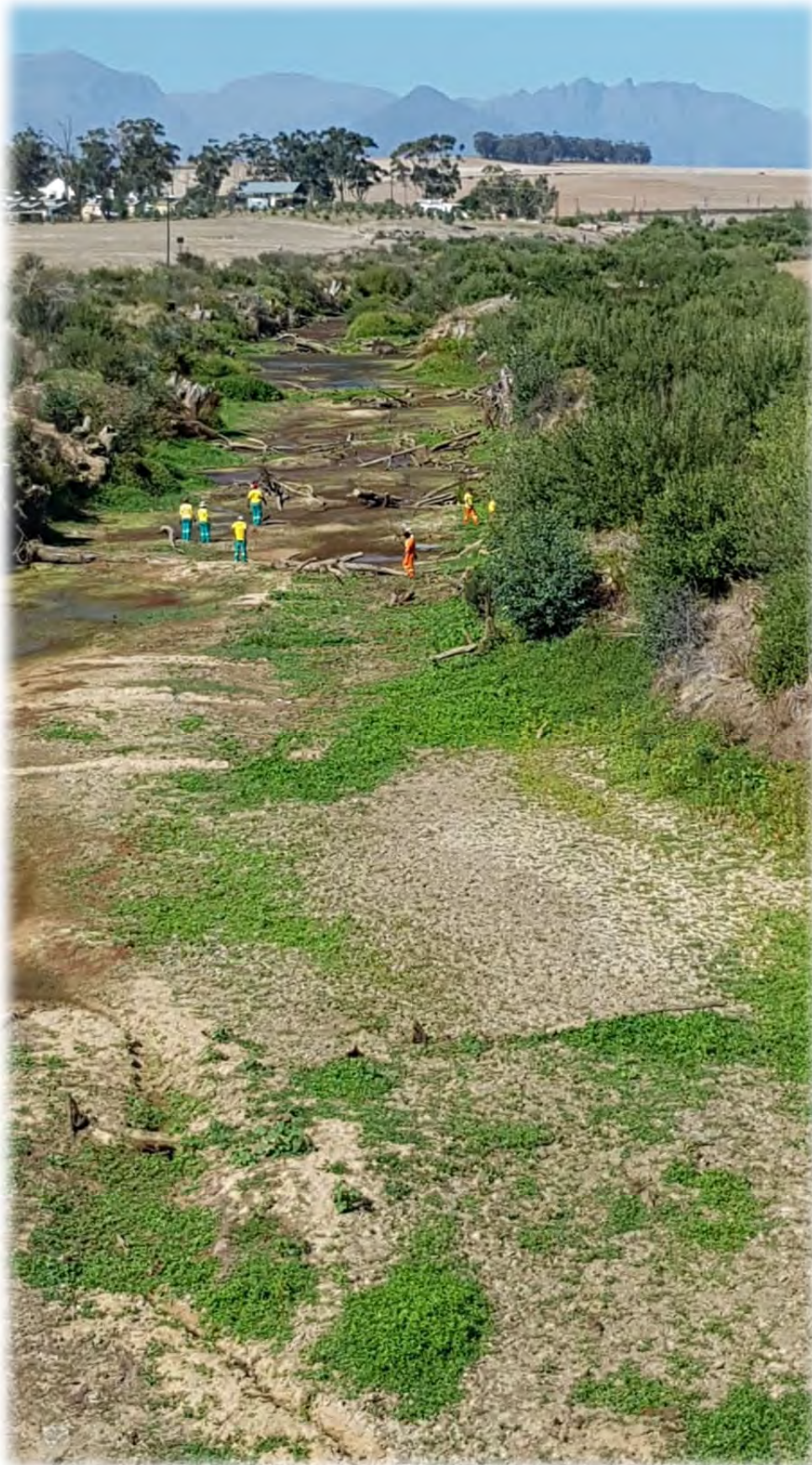
Figure 10: The EPW programme was utilized to the fullest by appointing volunteers to sweep the area along the river by clearing unnecessary rubble and obstacles in anticipation of the flow 5 hours ahead
